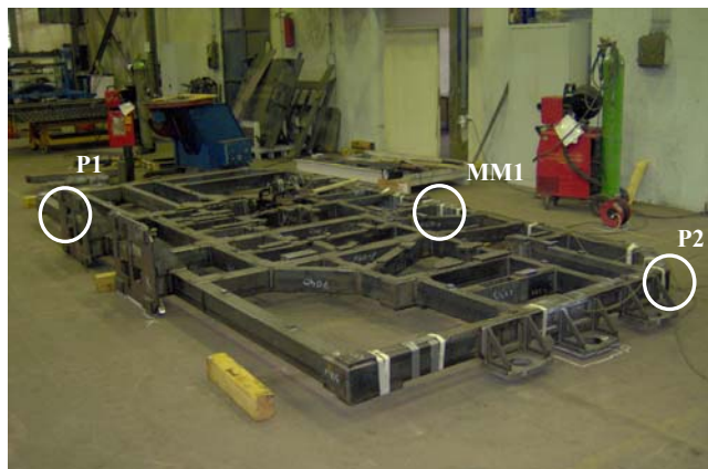
Figure 1. Treatment of the construction 1
