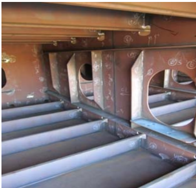
Figure 3. The inner space of the central section double bottom ballast spaces
