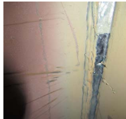
Figure 4. Weld between plates
