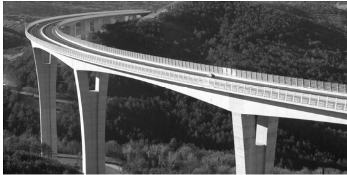
Figure 1. The view of the viaduct Crni Kal
